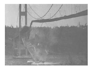
[Peter shows a film of the bridge oscillating. When the twisting motion was at the maximum, elevation of the sidewalk at the right was 28 feet (8.5m) higher than the sidewalk at the left.]
